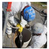
The necessary safety measures must be observed during insertion of the elements into the manhole. It is recommended to use a small crane to lift all panels inside.
