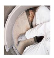
After installation of the berm elements, one can easily install the DURA.Port ring segments on top for the full remaining height of the manhole. Each row needs to be aligned on the folded joint contact surfaces of the previous row and glued to the existing structure to ensure the watertightness of the system.
