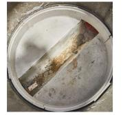
3. Repeat the alignment with the precut elements and again set up the first row of segments (if necessary with wedges or spacers against the old manhole wall to fix them in place). Make sure that the vertical joints of the segment elements do not sit above an inlet or outlet, if possible.
