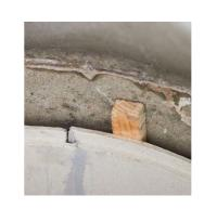
Spacers or wedges can be used between the existing wall and the new elements to align the panels correctly.
