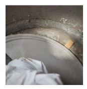
To verify the alignment, it is recommended to enter the 10 cm vertical DURA.Port ring segment elements in the manhole and place them in the folded joint as a way to easily check the alignment. The alignment is correct if a complete circle can be created with the ring of DURA.Port elements.
