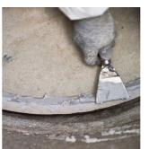
All joints between the ring segments shall be connected with DURA.Glue to ensure a watertight and robust system. Before applying the DURA.Glue, care must be taken that the area where the glue will be applied is dust-free.
